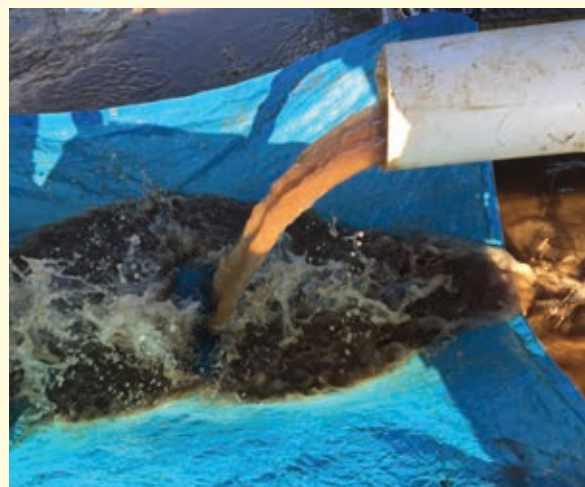
Discolouration of water during well servicing indicating removal of solids from screen section.
