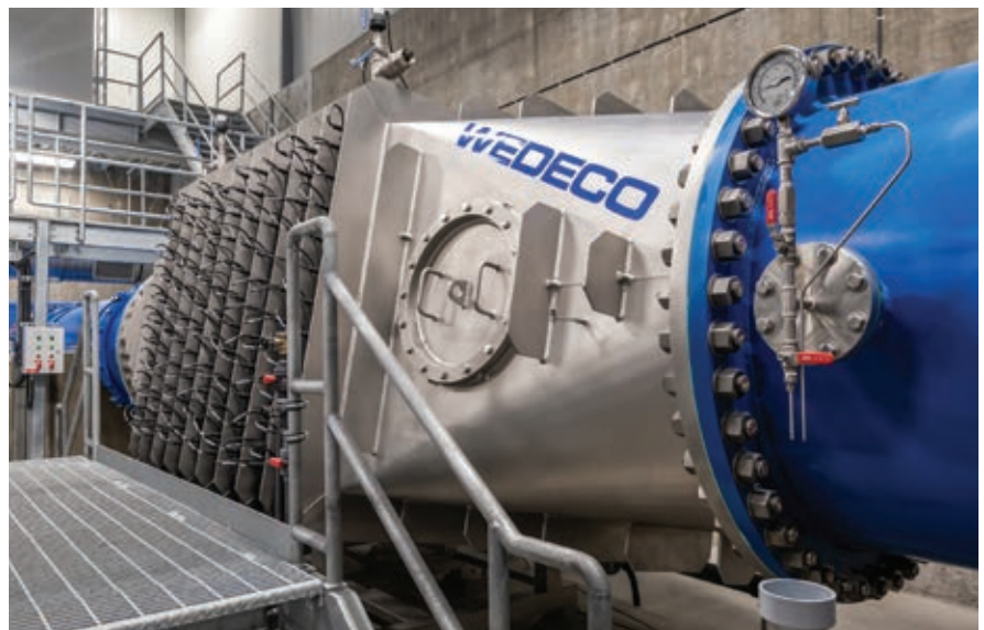
The operations platform with the UV reactor orientated to facilitate UV lamp removal and maintenance.
