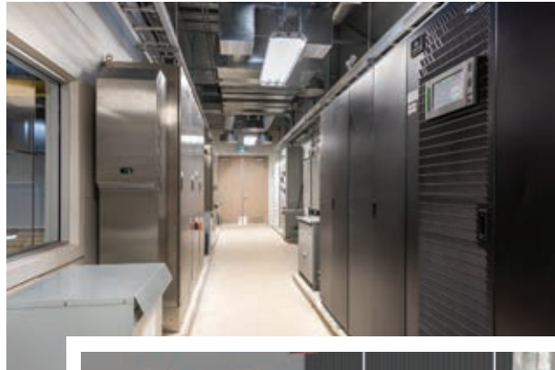
Figure 1. The 350kW uninterruptible power supply equipment and UV controls.
