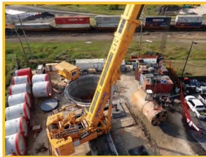
Launch of DECAST microtunnelling pipe.
