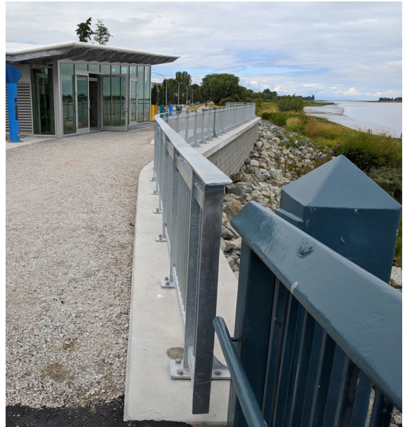
Dike upgrades along the foreshore were specifically designed to keep all disturbances above the high water level, helping to preserve the natural habitat.
