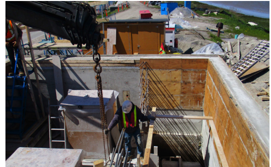
The existing wet well structure was successfully incorporated into the design.
