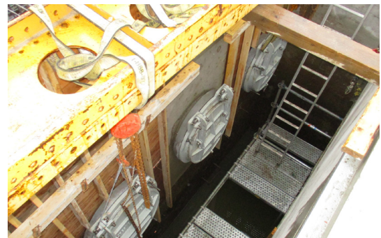
Construction of the pump discharge gates, located in the floodbox.
